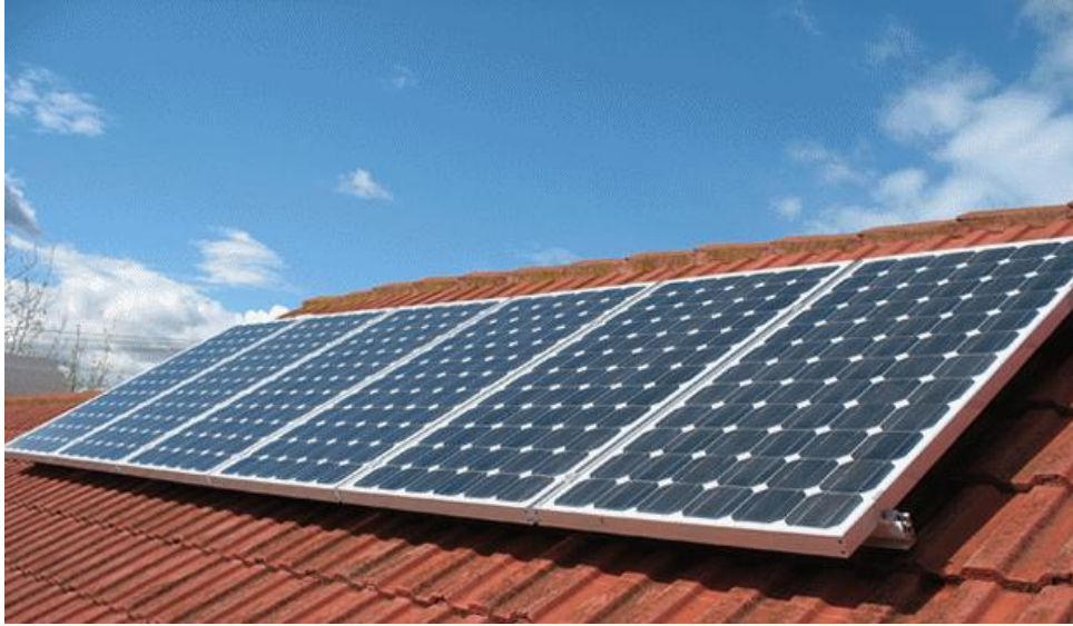
Picture 59: Solar cells on the roof of a house
